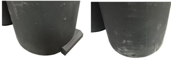
Before and after battery foot removed
