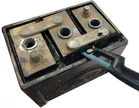
Hacksaw cutting the battery connections
