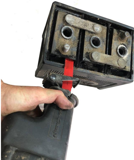
Sawzall makes quick work cutting connections
